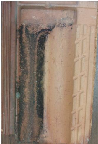
On the left side of this roofing tile can be seen the blackened area cause by mould and fallout. There is also spots evident of a lighter shade of a roundish fungal growth. These are normally very difficult to remove as they are 'growing' from the pours of the tile.
