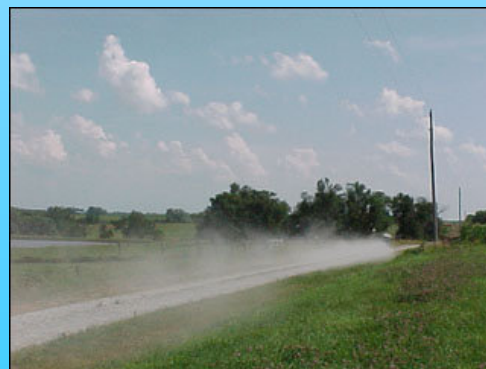
Fugitive Dust from untreated roads can produce tons of particulate matter causing air pollution problems.
